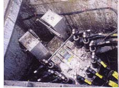
ElbowSense Current Monitoring Ring used in a Two Way Submersible switch.
