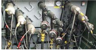
ElbowSense Current Monitoring Ring used in a Two Way Submersible switch.
