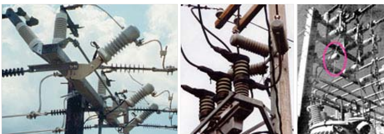
Substation/Switchgear style CVMI on air break and vacuum bottle switches and for SCADA in substations with 1% accuracy
